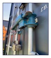
For further security, a special highsecurity Door Bar lock is installed. The features of this Lock are: The claws are forked and must be placed over the 2 door bar distance holders. The connecting bar, between these claws, are constructed of material that is resistant against drilling and flexing.
